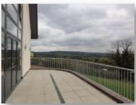
Figure 9: The existing raised deck in front of the hall has views across the open countryside
