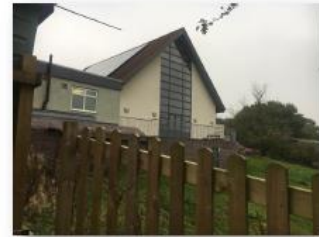
Figure 2: The new school hall – the land slopes steeply away from the building
