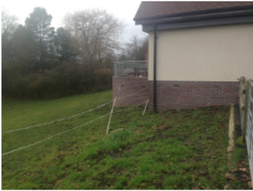
Figure 8: The proposed extension would continue level from the existing hall deck which would require steps and a ramp down to the ground level of the car park for access and escape.
