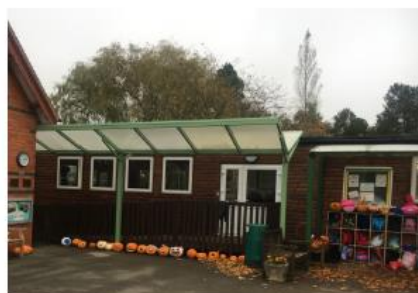
Figure 6: The double mobile is sited tight up to the existing school and occupies valuable hard play
