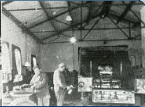
Mechanics at work in the service area
