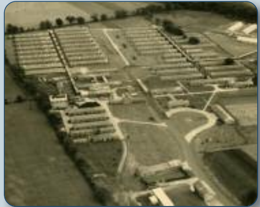
Aerial view of the newly constructed American Military Hospital at Malvern Wells.
