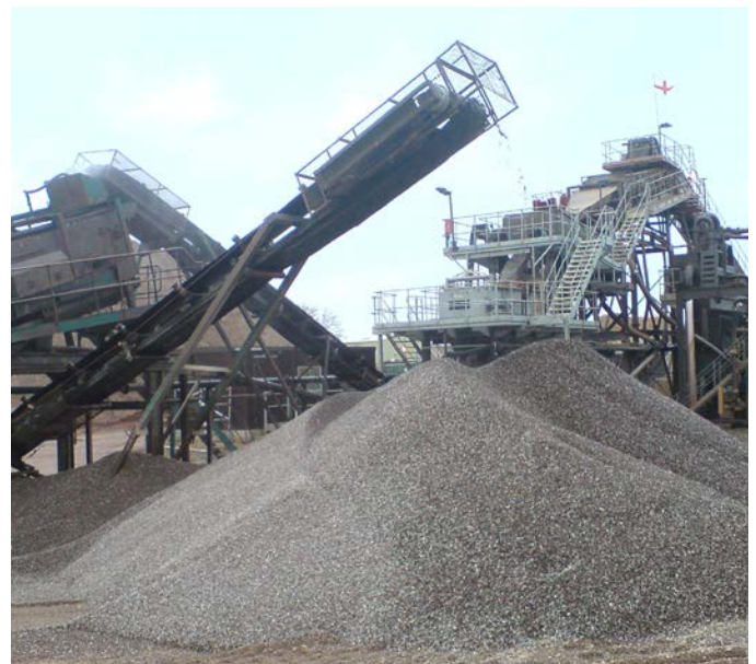
Processing plant at Ryall House Farm sand and gravel working
