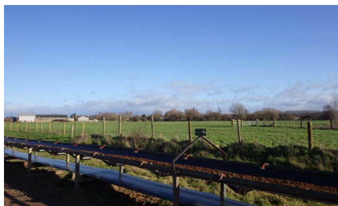
Conveyor at Clifton Quarry
