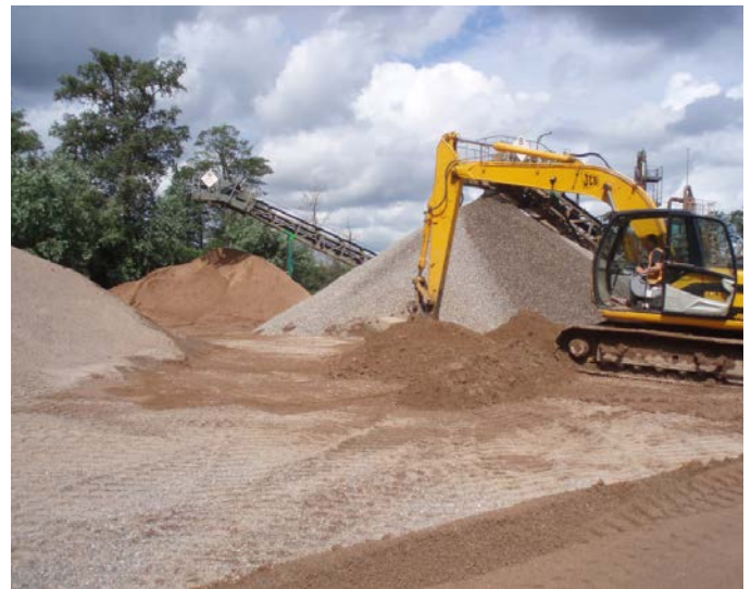
Processing at Clifton sand and gravel working
