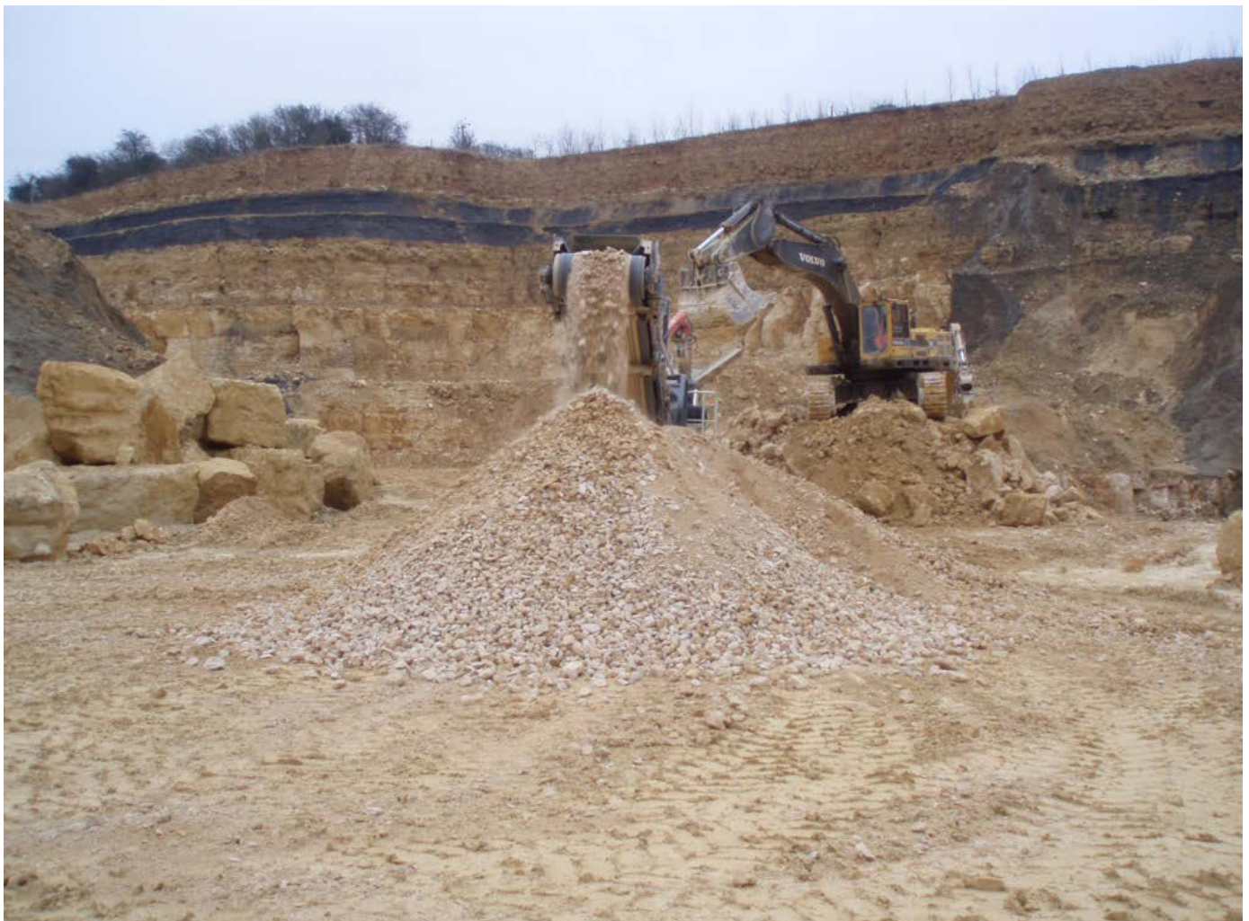
Processing crushed rock at Fish Hill Quarry
