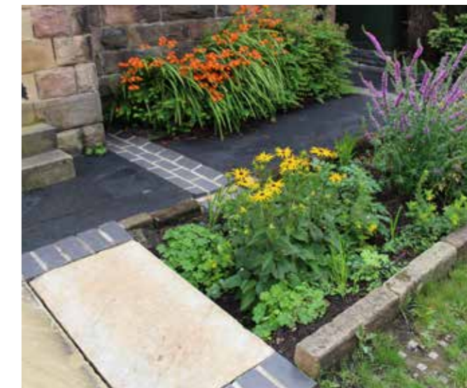
Strutts Centre, Belper. Brick channels collect roofwater for linear raingarden with garden style planting.
