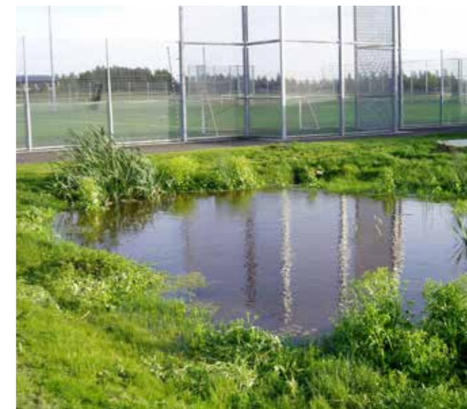
Pershore High School, Worcestershire. Swale conveyance into pond site control for final treatment and storage.
