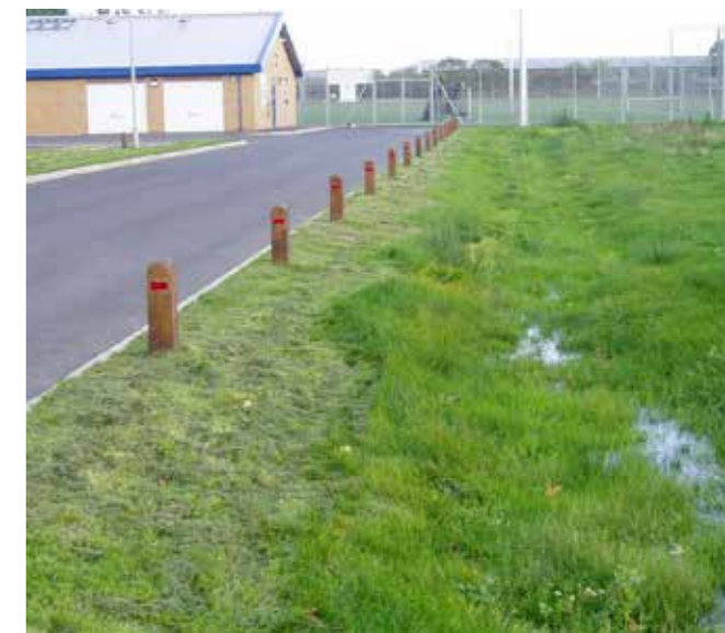
Pershore High School, Worcestershire. Low risk access road with 1.2m wide filter strip source control and conveyance swale.
