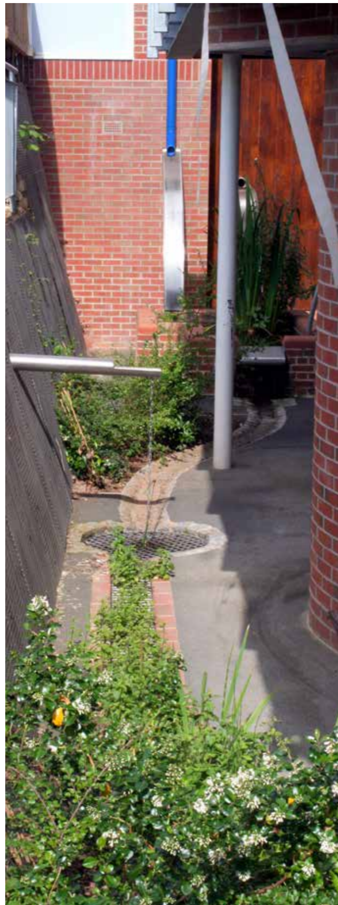
Fort Royal Primary School, Worcester. Mini-courtyard with rainchain, rain slide, raised pool and rill.
