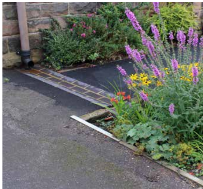
Strutts Centre, Belper. A retrofit downpipe shoe and brick channel into a raingarden.
