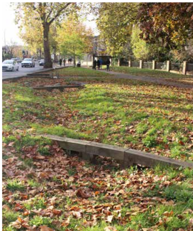
Rectory Gardens Rainpark, Hornsey. Forebays, swales and underdrained basins use SuDS turf (100-150mm) to filter runoff, with amenity grass for public use.
