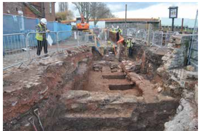
Construction of a flood alleviation scheme
