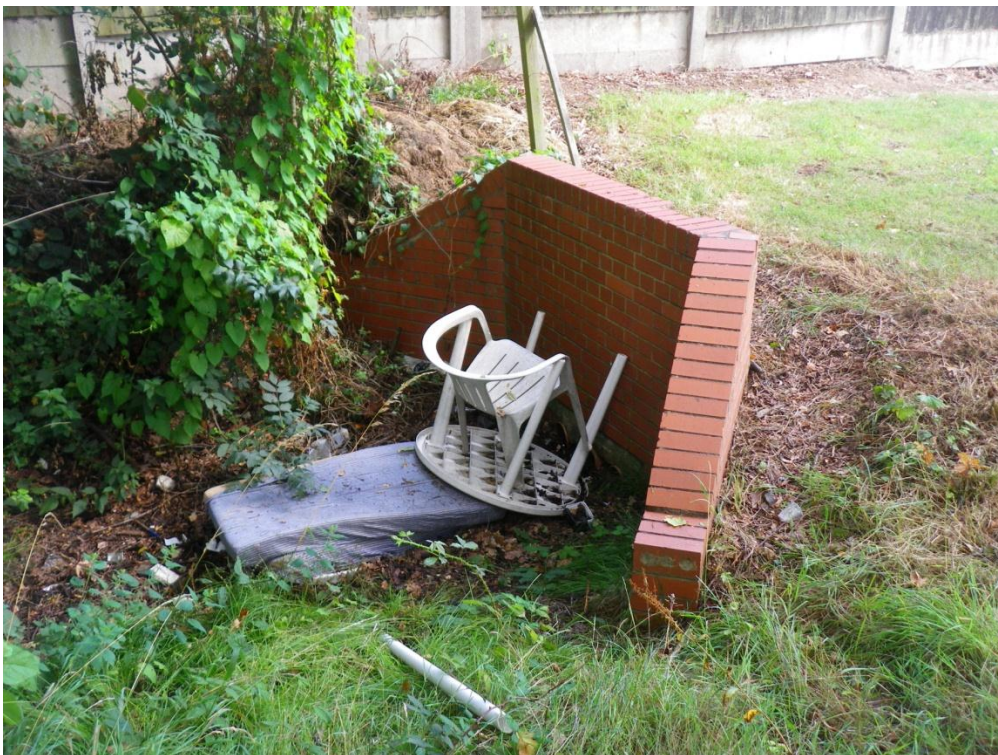
Photograph 6 - Entrance of culvert under Salters lane - Red Ditch
