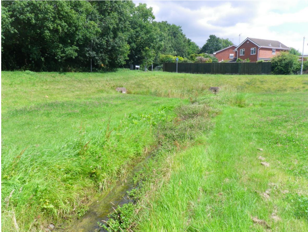
Photograph 19 - Attenuation area control structure, Church Road, Webheath
